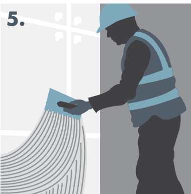
5. Applying notches within basecoat.
